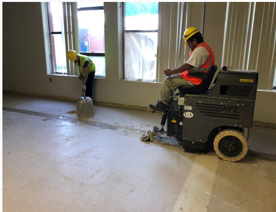
Removal of flooring in classroom building
