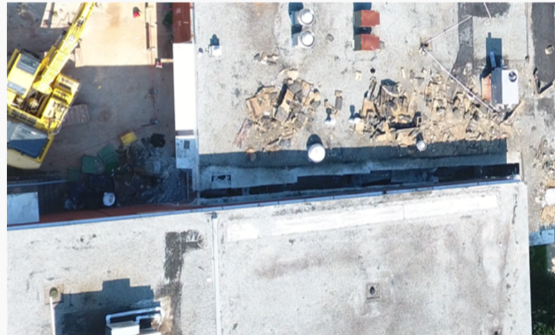
Separation of buildings schedule for demolition
